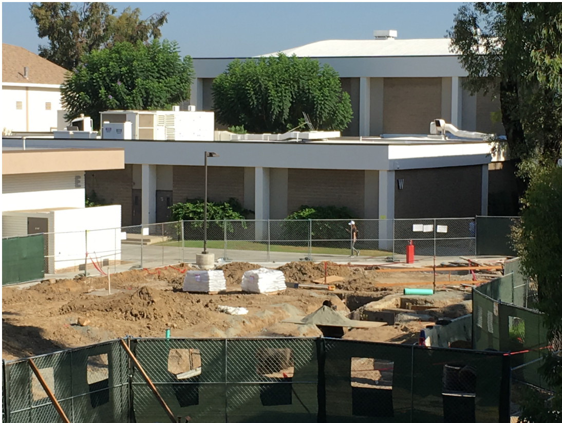
Phase 4 Construction Zone
