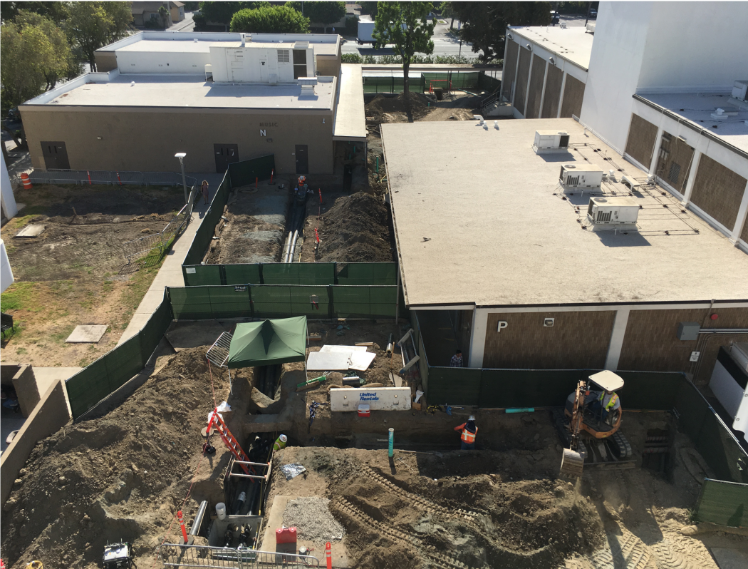
Phase 3 Construction Zone
