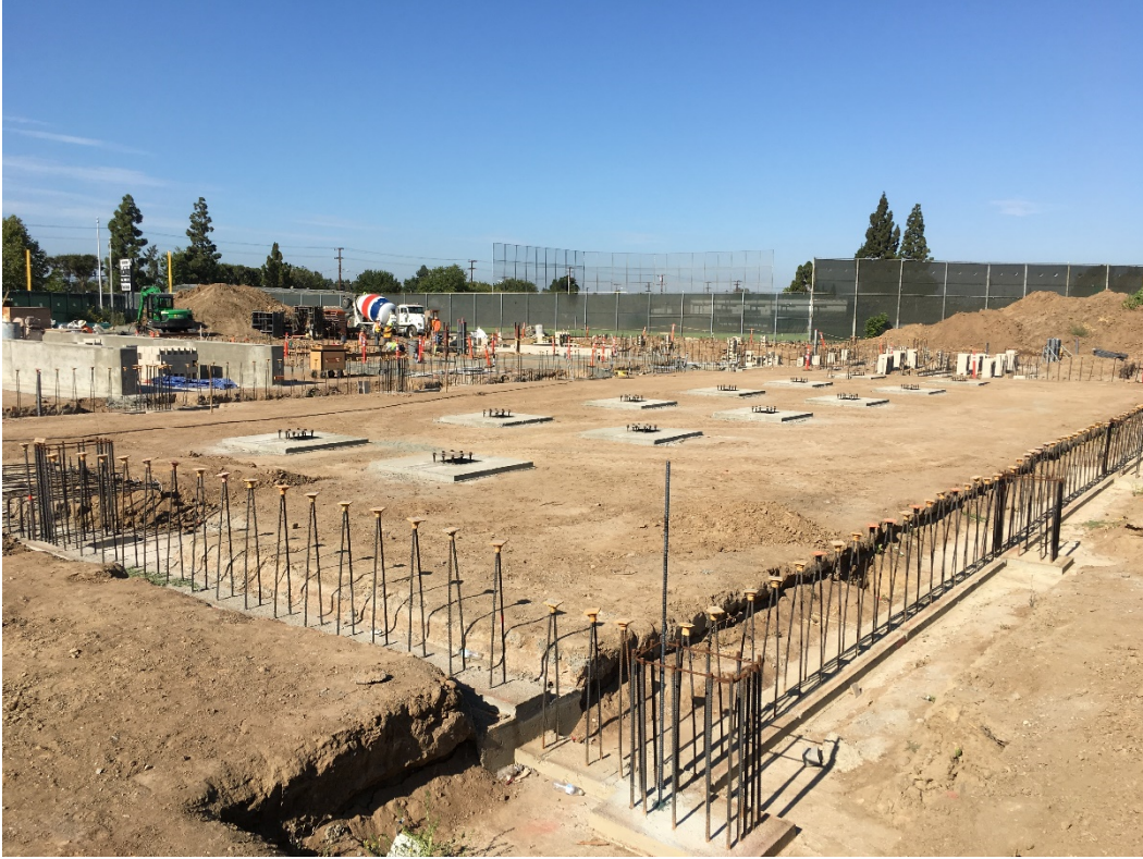
Central Plant Construction Zone
