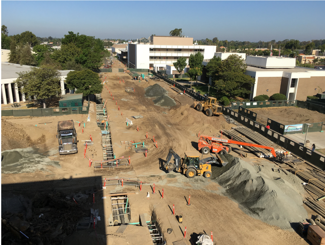
Phase 4 and 5 Construction Zone
